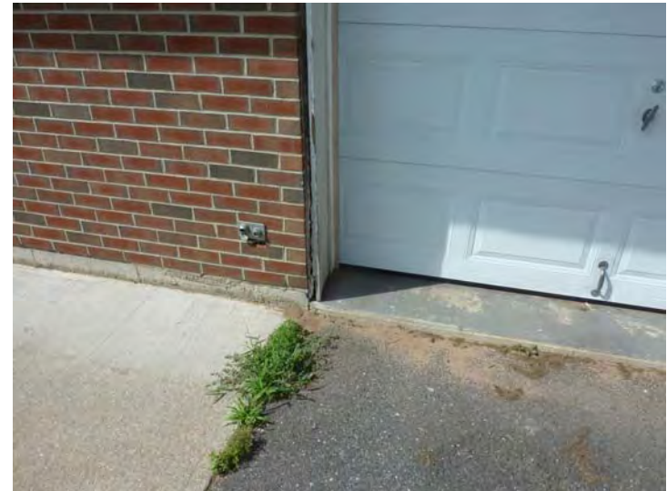
Typical failure at garage door trim is shown to be repaired in Year 1.
