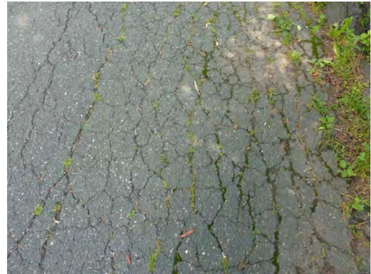
Typical sub-base failure of asphalt paving in development driveway. Overlay of asphalt paving is shown in Year 1.
