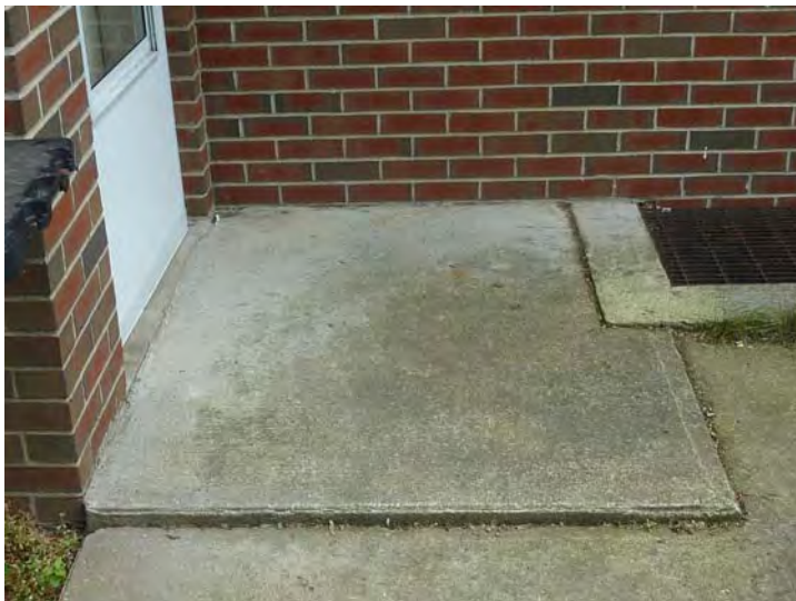
Typical trip hazard at concrete unit stoop. All trip hazards are shown to be eliminated in Year 1.
