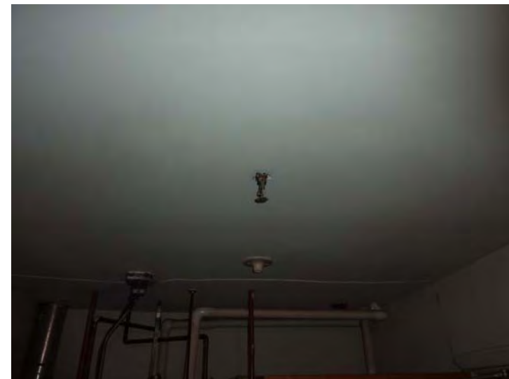
Residential sprinkler in first floor Mechanical Room with washer/dryer, gas-fired boiler and domestic hot water heater in 2-bedroom apartments.
