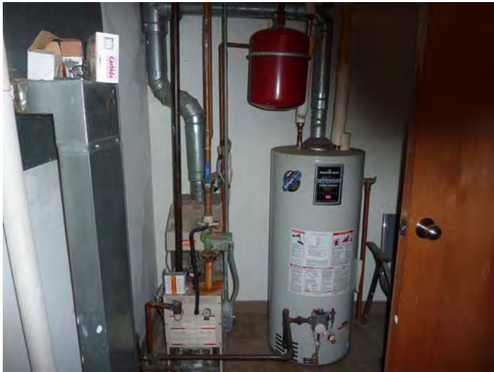
Gas-fired boiler and domestic hot water heater in first floor Mechanical Room in 2-bedroom apartments.
