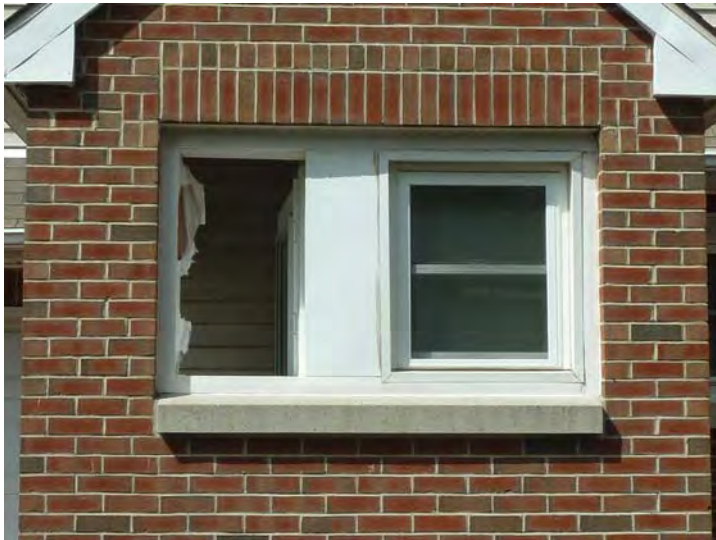
Missing window at unit entry to stair is shown to be replaced in Year 1.
